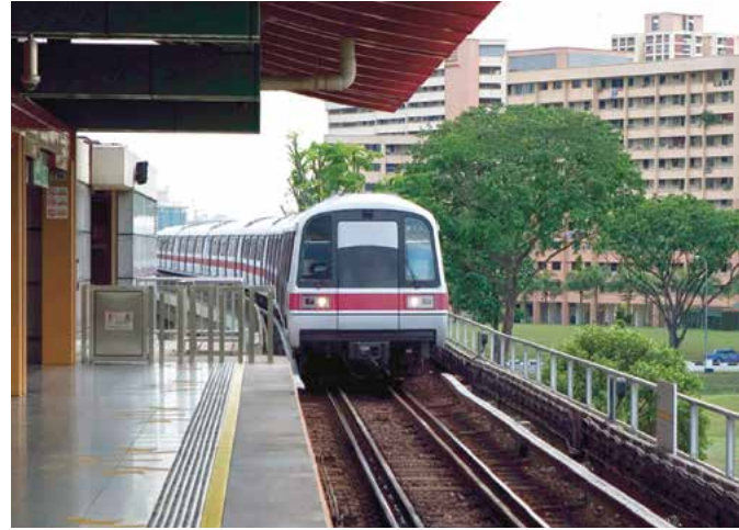
Circle Line, Mass Rapid Transit System, Singapore.
